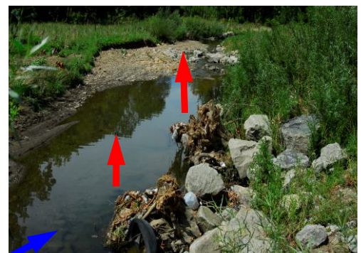
Root Wads Causing Bank Failure
