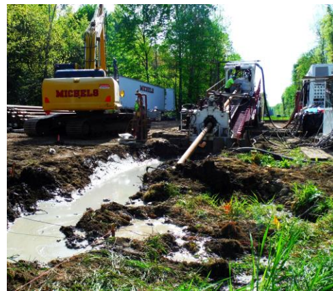
Direction Drill Rig
