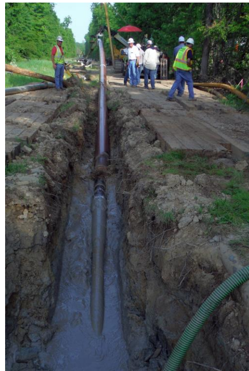
Replacement pipe pullback
