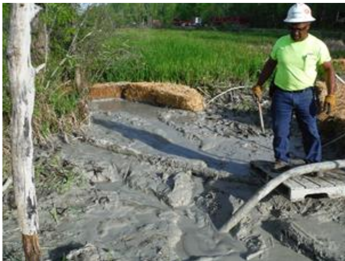
Inadvertent Return Cleanup
