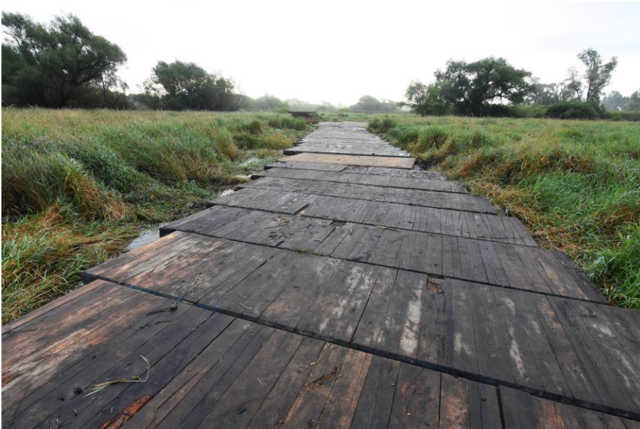
Composite timber mat road through wetland
