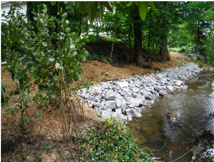
Constructed LPSTP looking upstream
