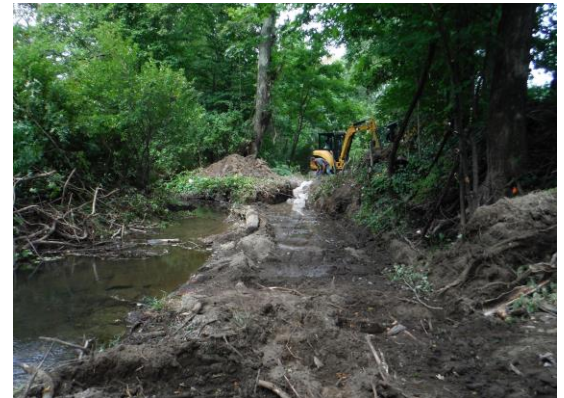
Trout Run prior to LPSTP installation (bank failure to right of stream channel)
