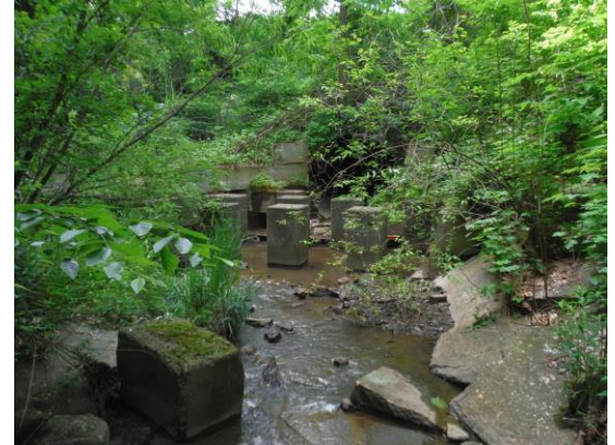
Scott Run Culvert Outlet
