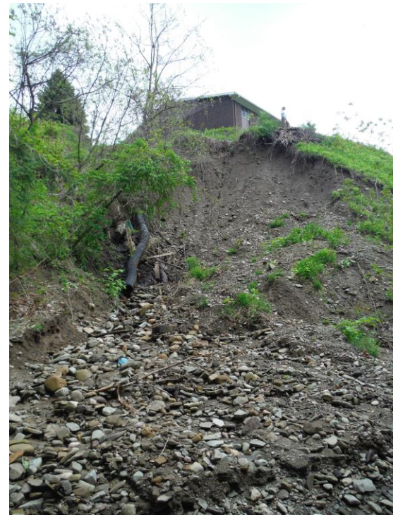
Large Bank Failure
