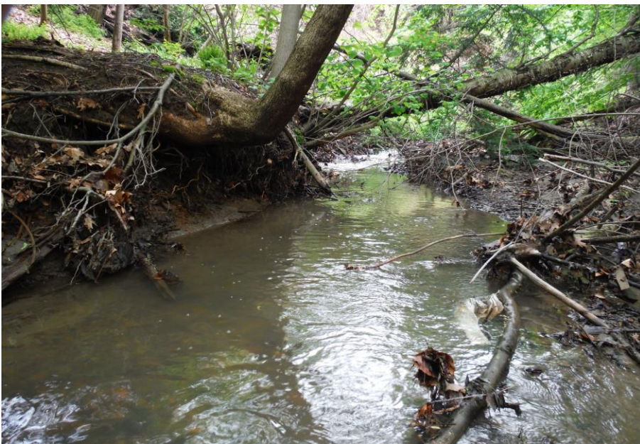
Channel Degradation from Urban Stormwater Flows
