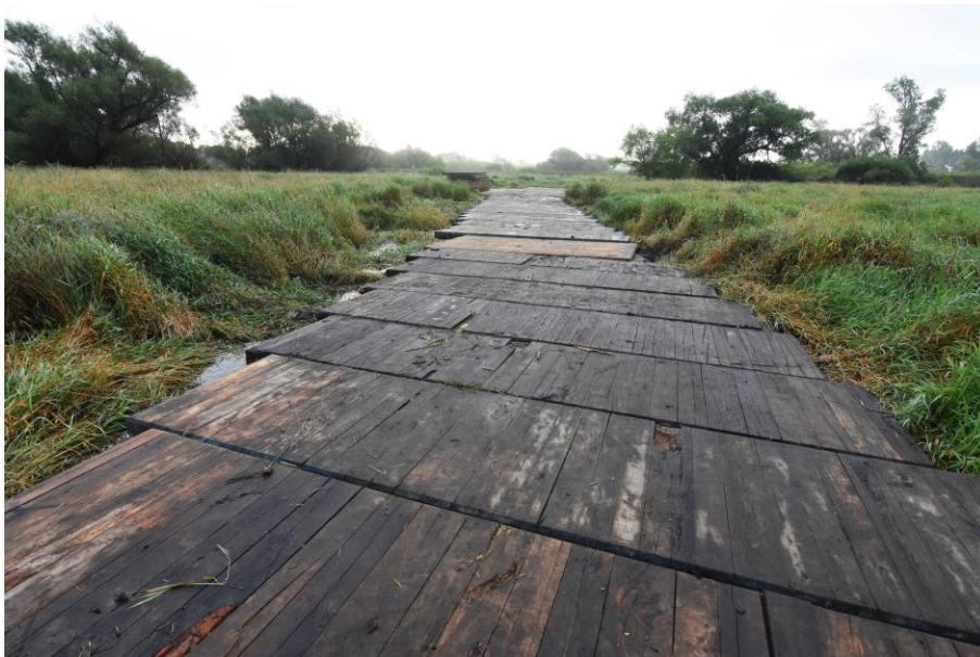
Composite timber mat road through wetland
