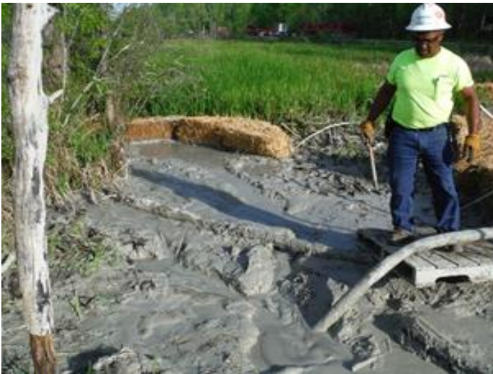
Inadvertent Return Cleanup
