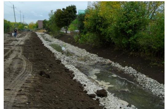
Newbury Rock Riffles Under Construction
